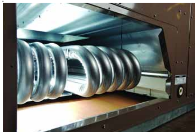
Figure 16: Bottom Supply Opening For Side Duct Conversion
