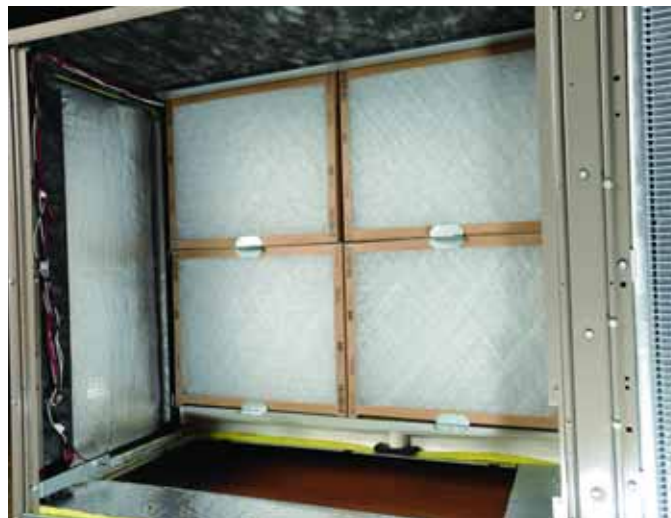
Figure 15: Bottom Return Opening For Side Duct Conversion
